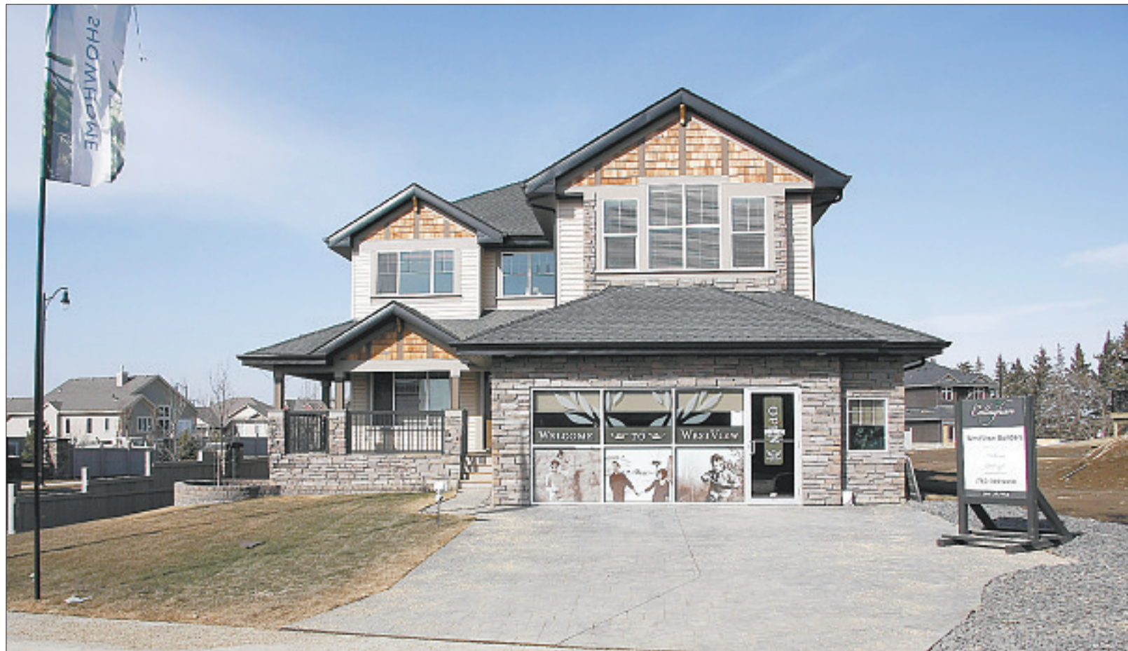
The show home for Westview Builders is pictured above. The company is one of five developers represented in the Callaghan community.
